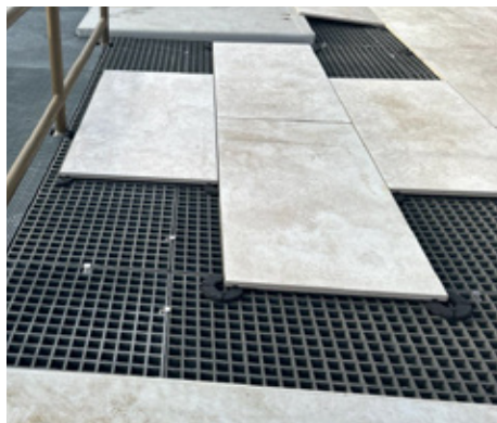
Porcelain paver installation using MacroMesh FRP grating support and rubber spacer pads.
