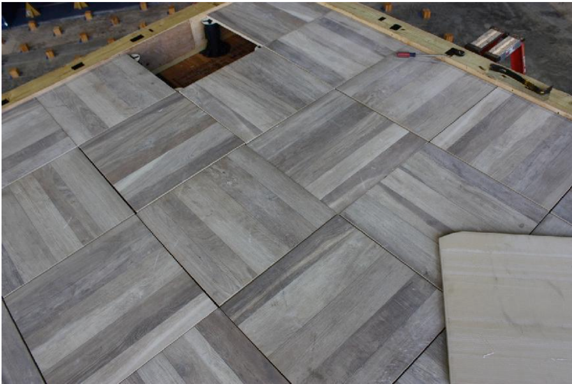
Figure 14 - Porcelain paver blown off by the wind from its location along the perimeter of the windward edge of the roof. A chipped corner may be seen on the paver from when it hit down.
