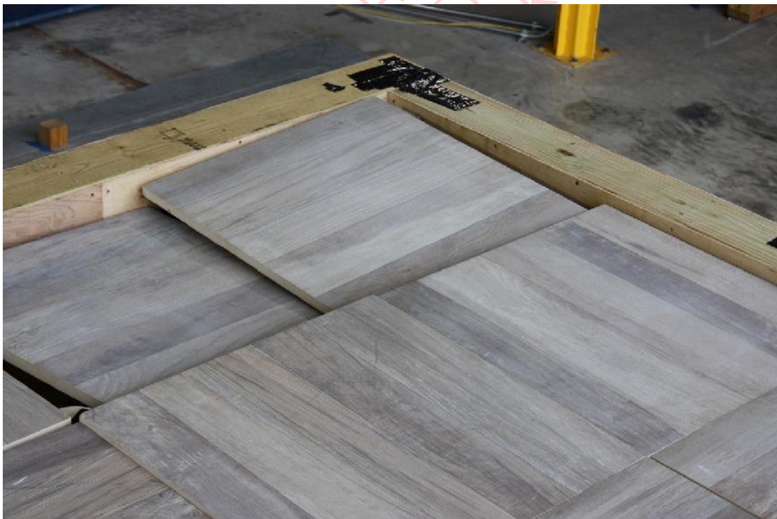
Figure 15 - Pavers pushed down into the windward corner of the roof by the wind.
