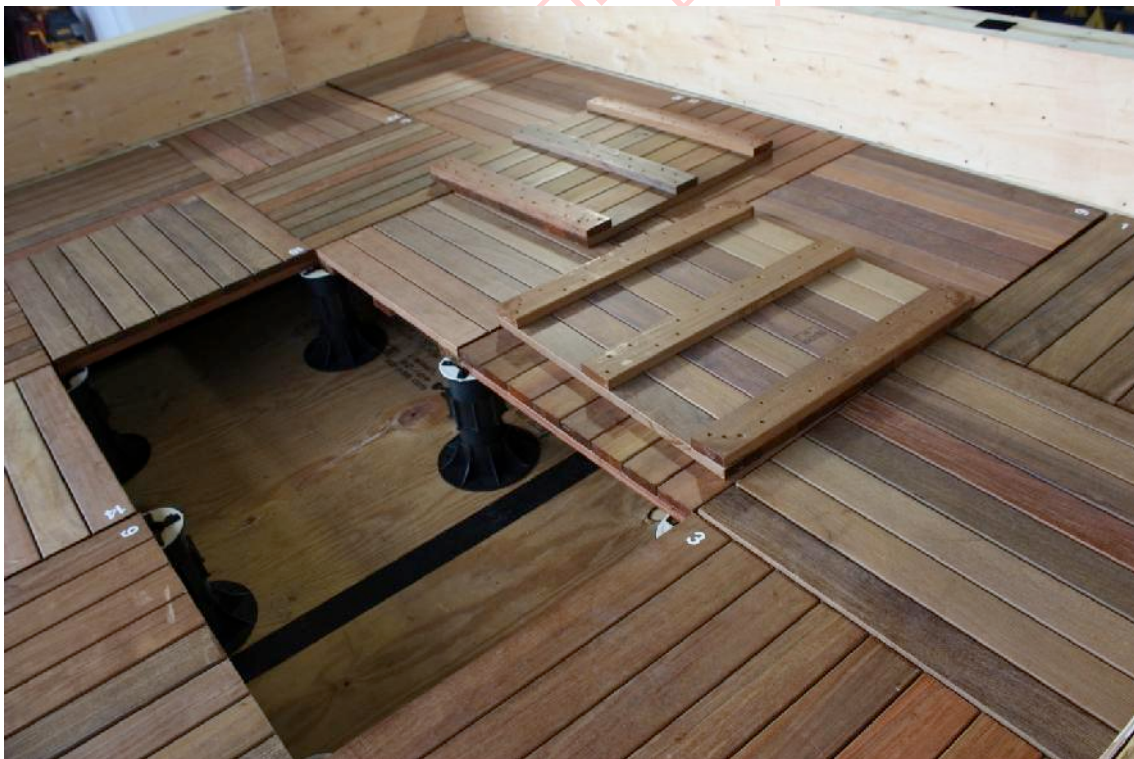
Figure 9 - Wood pavers laid out in basket wave configuration. The 2 pavers were flipped upside by the wind. Pavers were flipped in the direction of the oncoming wind.
