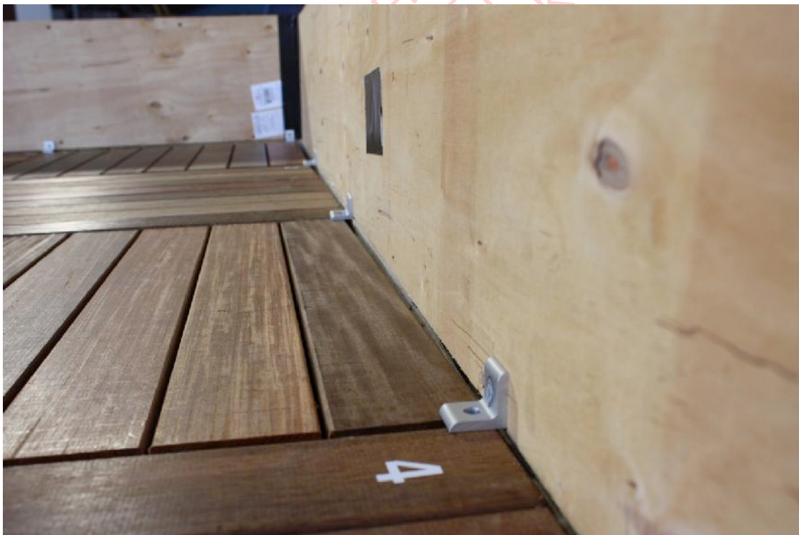
Figure 11 - Detail of the perimeter paver locking devices
