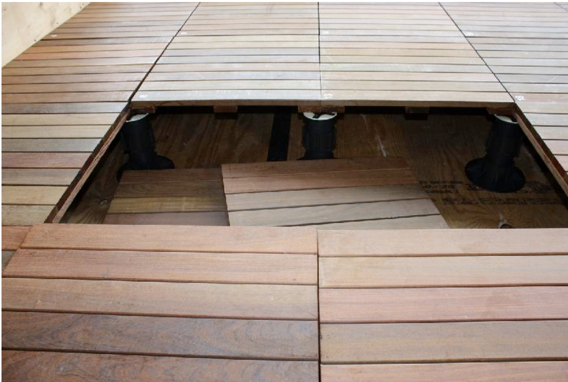
Figure 6 - Pavers blown off pedestals; wind picked them up but didn't blow them off the roof. As they set down they fell onto the roof deck pushing away some of the adjacent pedestals
